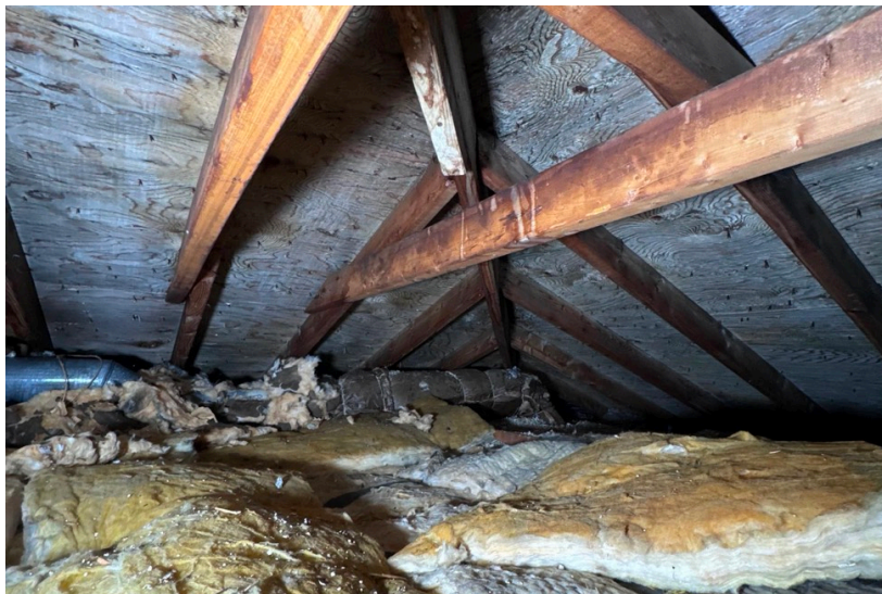
Glaswol tussen houten dakspanten. Foto: Canada's Restoration Services, Unsplash.
